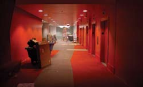
Journalism Department elevator bay during construction, summer 2005.
